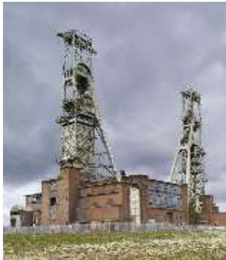
Clipstone Colliery, Nottinghamshire, a state of the art post-war deep mining facility with 213ft high headframes.
