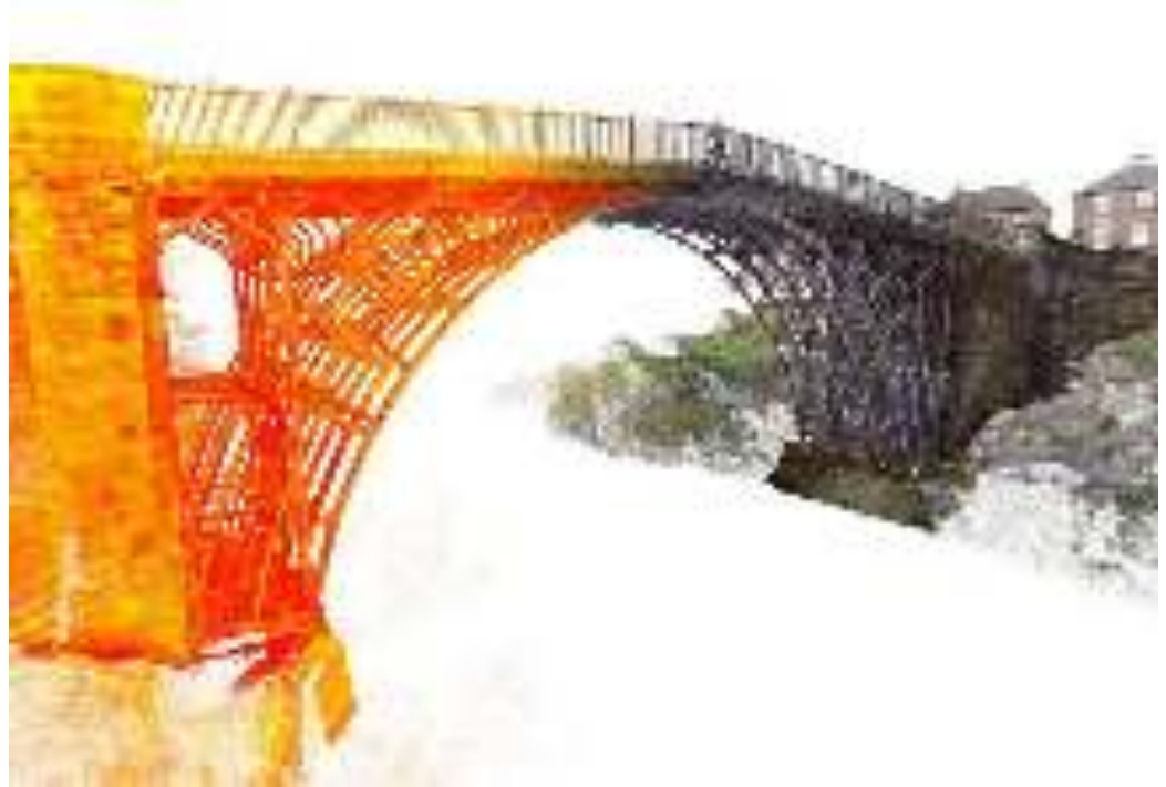
The Iron Bridge - showing a representation of the laser scan data that was captured in 2012 and contributed to the current investigation, repair and conservation of this iconic industrial monument.
