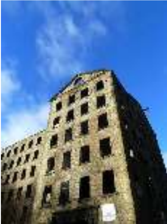
Left: Grade II* Rawson's Mill, Calderdale, Yorks, also known as Old Lane Mill was built for James Ackroyd in 1825-28. It is the oldest and largest surviving example of a multi-storey, steam powered, iron-framed textile mill and has been derelict for decades. Right: Derelict mill in Rochdale, Greater Manchester.
