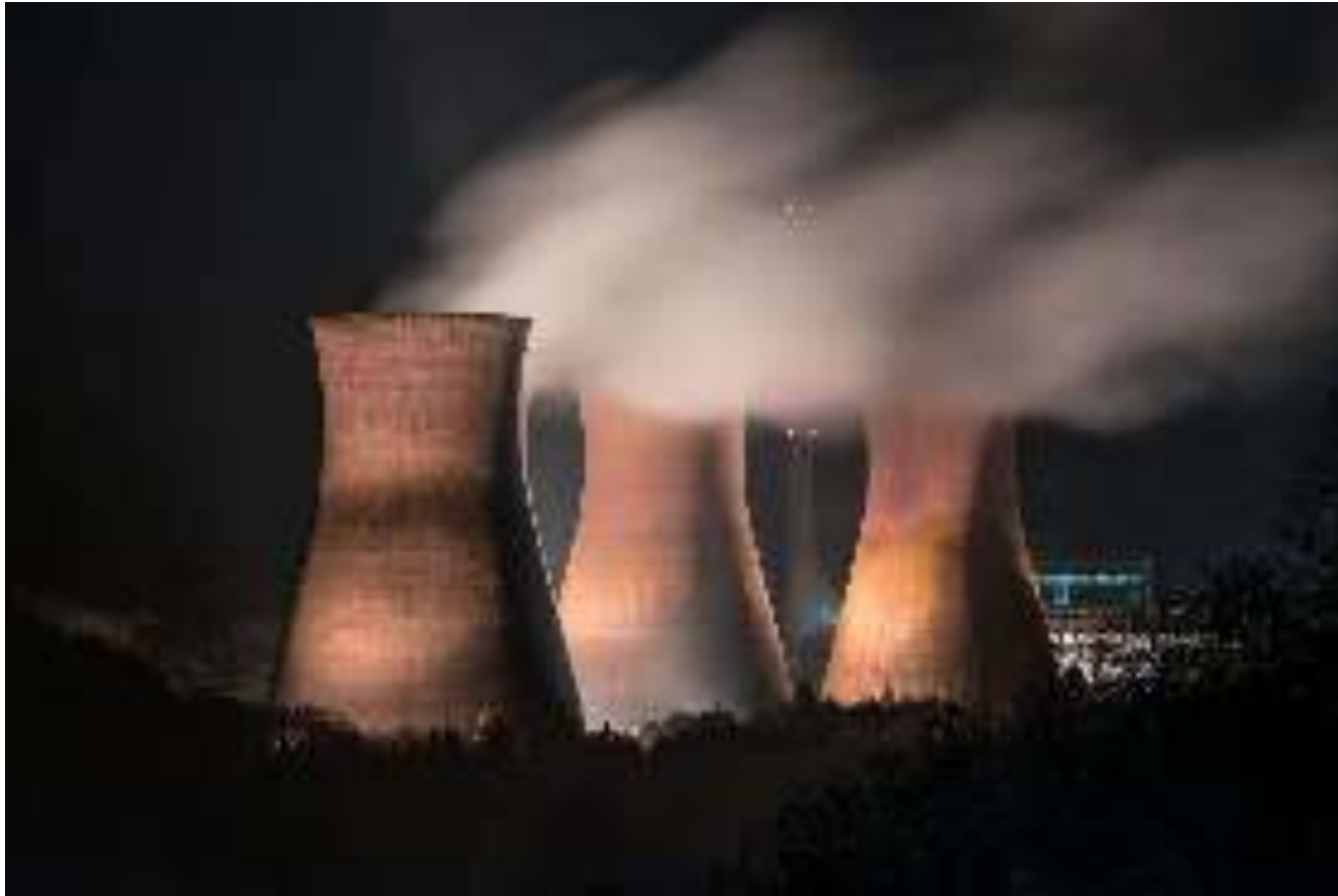
Power Stations - Ironbridge Power Station, Buildwas Road, Telford, Shropshire
