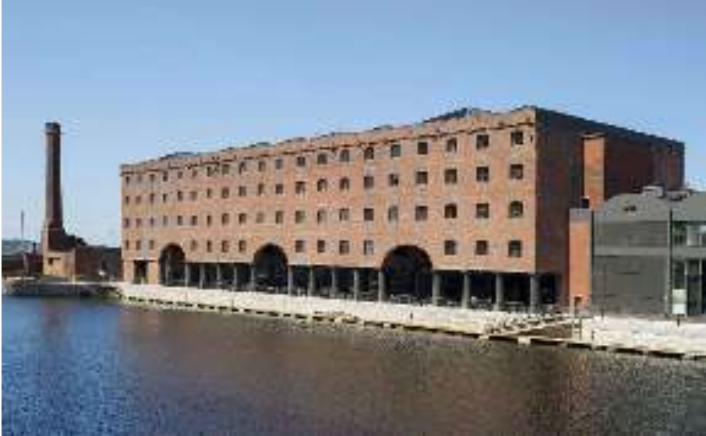
The converted North Warehouse, Stanley Dock, incorporating the new Titanic Hotel, Liverpool WHS.
