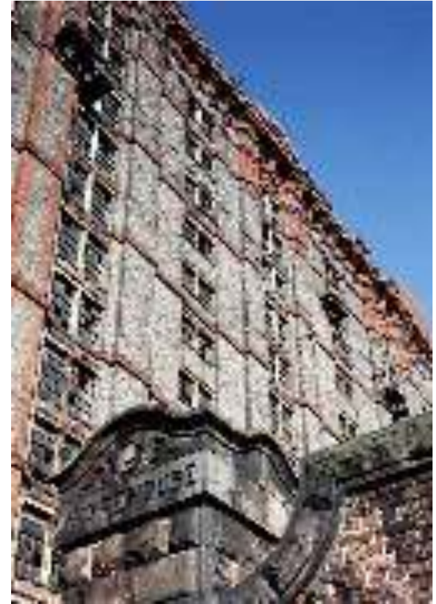
The huge Tobacco Warehouse, Stanley Dock, Liverpool, being converted to 538 apartments.
