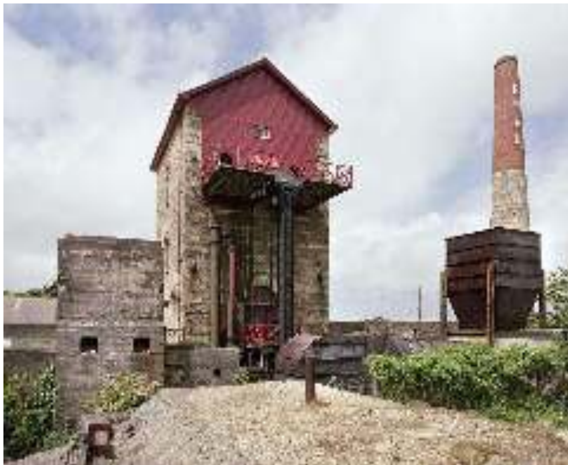
Taylor's Shaft pumping engine house and chimney from the south west, East Pool mine, Cornwall, Cornwall and West Devon Mining Landscape WHS.
