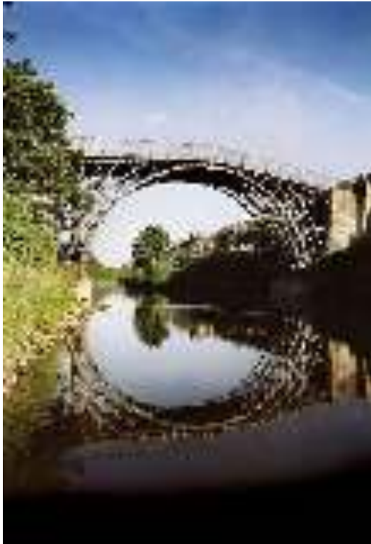
Iron Bridge, Shropshire by Abraham Darby III. The world's first major cast-iron bridge opened in 1781 is at the heart of an industrial landscape comprising 36 listed or scheduled structures.
