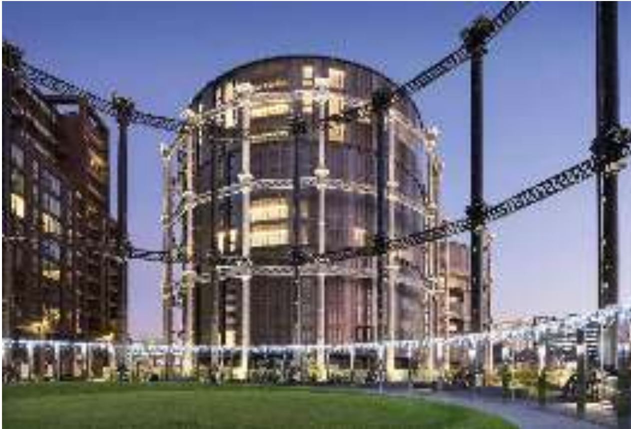
Former Gasholders, Gasholder Park, Kings Cross, Camden, London. General twilight view of gasholders No 8, 10, 11, 12, refurbished by Wilkinson Eyre Architects .
