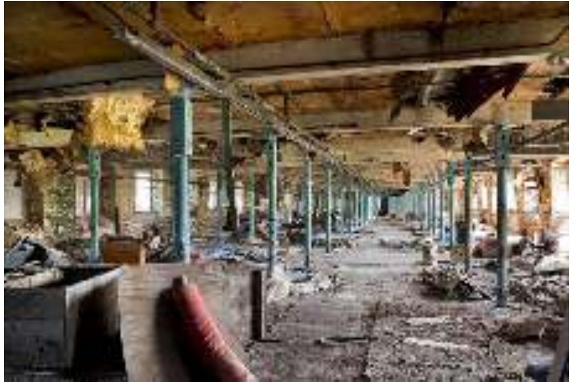
Left: Grade II* Rawson's Mill, Calderdale, Yorks, also known as Old Lane Mill was built for James Ackroyd in 1825-28. It is the oldest and largest surviving example of a multi-storey, steam powered, iron-framed textile mill and has been derelict for decades. Right: Derelict mill in Rochdale, Greater Manchester.
