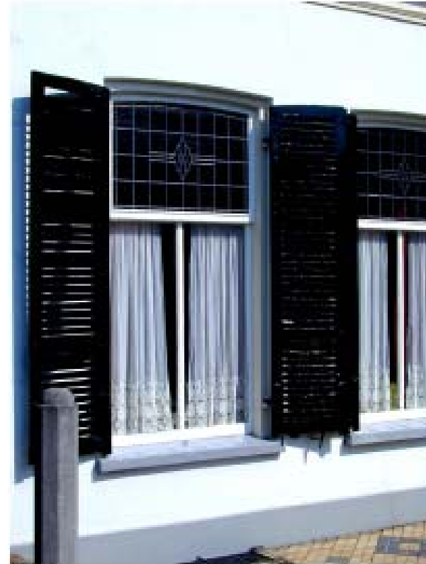
Shutters and venetian blinds can play an important role in controlling the indoor climate. A 19th-century example of lowered blinds.
