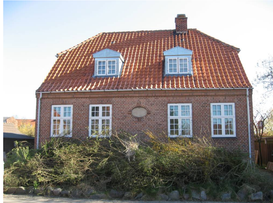
After energy renovation
