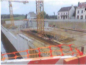
Next, side walls were built with a concrete coating before the installation of foundations, the construction of interior walls, support columns and the construction of a storm basin that can accommodate about 200 m<sup>3</sup> of water for supply to the bathrooms on the site.
