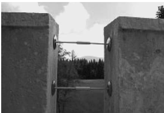
Fig. 20: Non-intrusive steel stoppers at terrace parapet.
