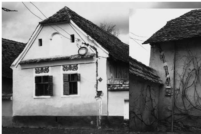
Fig. 23: Saxon house in conservation area, with meter on the street facade and (inserted) with the final solution of the meter in the courtyard facade. © MET, Transylvania.
