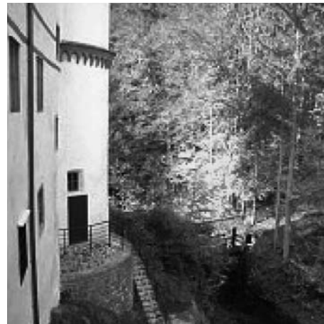
Fig. 19: Due to fire regulations, new terrace and steps down from tower gate have been built.
