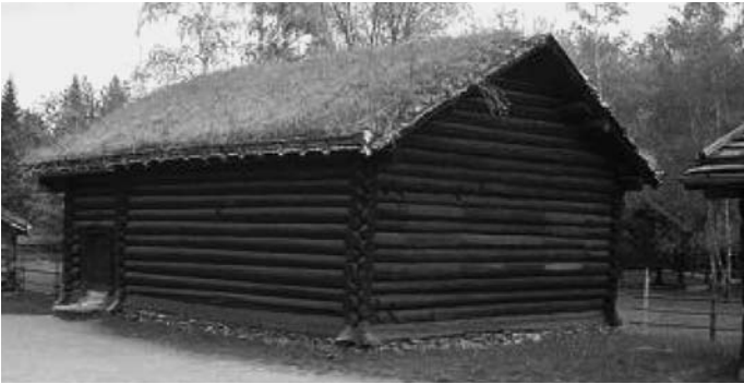
Fig. 15: Raulandsstua, log building from 1300, Norwegian Folk Museum. One of the oldest buildings of the museum, treated with wood-tar. Foto: Jan Anderssen.
