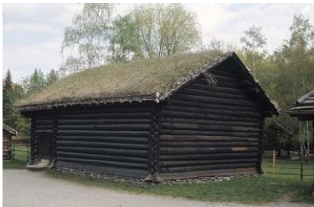
Above left: 2007 advertising for tradition log cabin. Above right: Advertising for contemporary dwelling. Photos: from advertising brochures. Bottom: Raulandsstua, log building from 1300, Norwegian Folk Museum. One of the oldest buildings of the museum, treated with wood-tar. Foto: Jan Anderssen,
