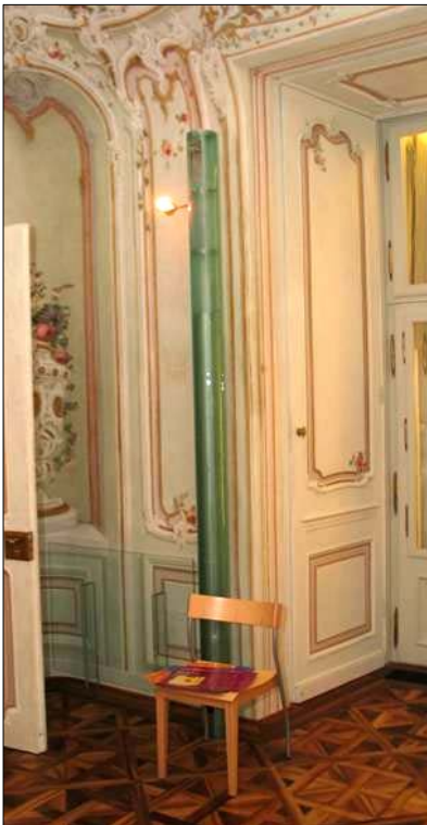
Picture 4: Purpose designed service column in Schönbrunn Palace
