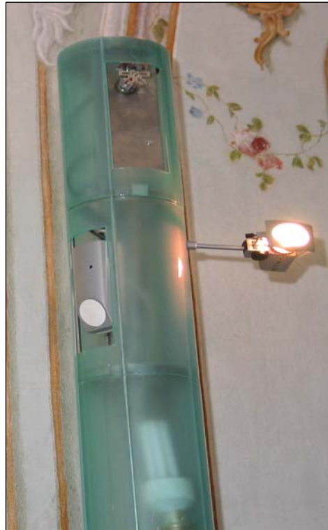
Picture 5: Purpose designed service column in Schönbrunn Palace detail
