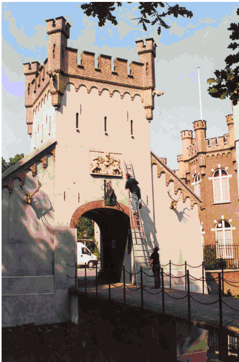
Stapelen castle Boxtel ,2005 NL. Traditional ladders can also be used instead of prescribed scaffolding. Note the man securing the ladder at ground level. Secure working is one of the major issues during the work of the inspectors. © Monumentenwacht Noord-Brabant
