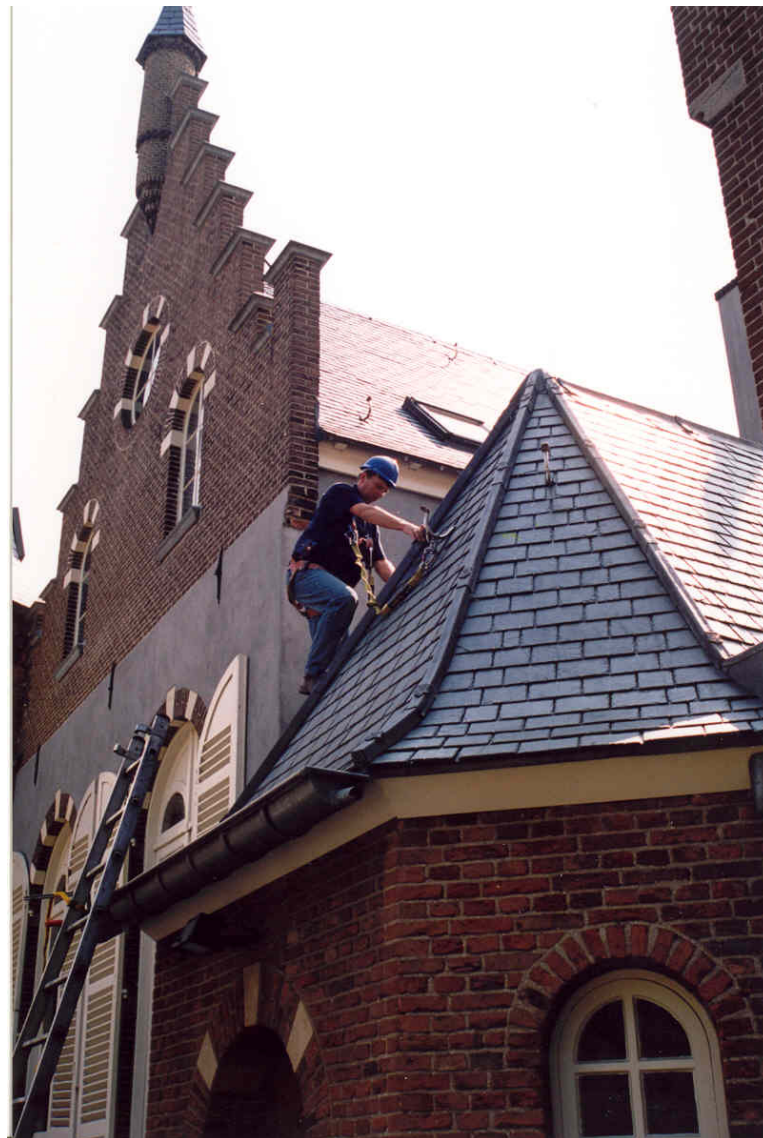
Stapelen castle Boxtel, 2005 NL Roof inspection for damages, using climbing safety gear and ladders. During the inspections, small-scale repair work might also be carried out by the inspectors. © Monumentenwacht Noord-Brabant
