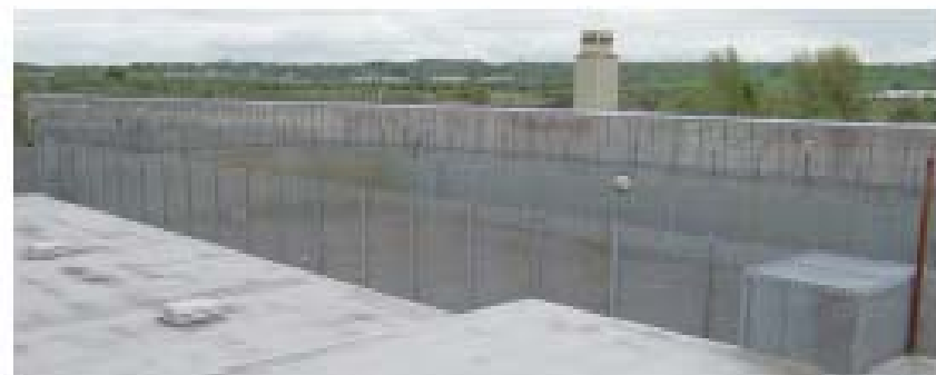
H6 southwest exercise yard, view from roof
