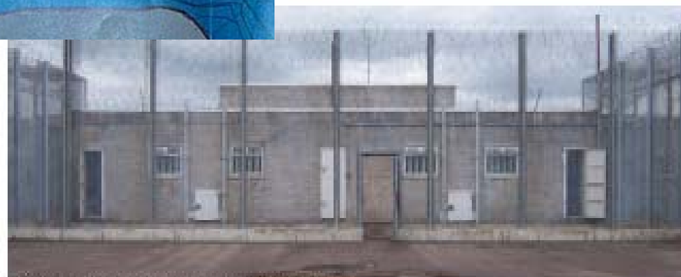
H6, south central elevation (external wall of filtration blocks)
