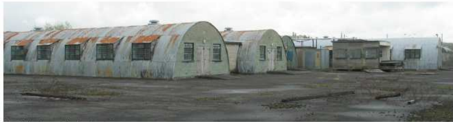
General view, Compound 8, view from northwest corner
