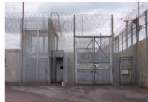
H6 southeast wing, end air lock, view from exercise yard
