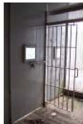
H6, entrance to passage to exercise yard, end of southwest wing
