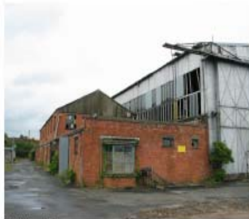
Building B-8, west range
