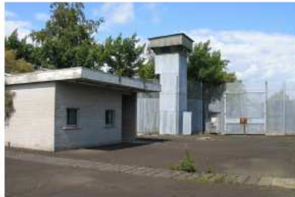
Building B/40 with B/21 behind
