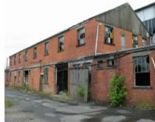
Building B-8, two storey section of west extension
