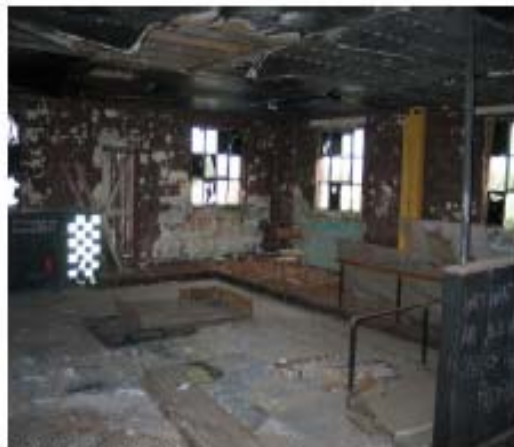
Building B-8, 1st floor bar area to the southwest
