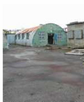
Building E8/4 from west with E8/3 behind
